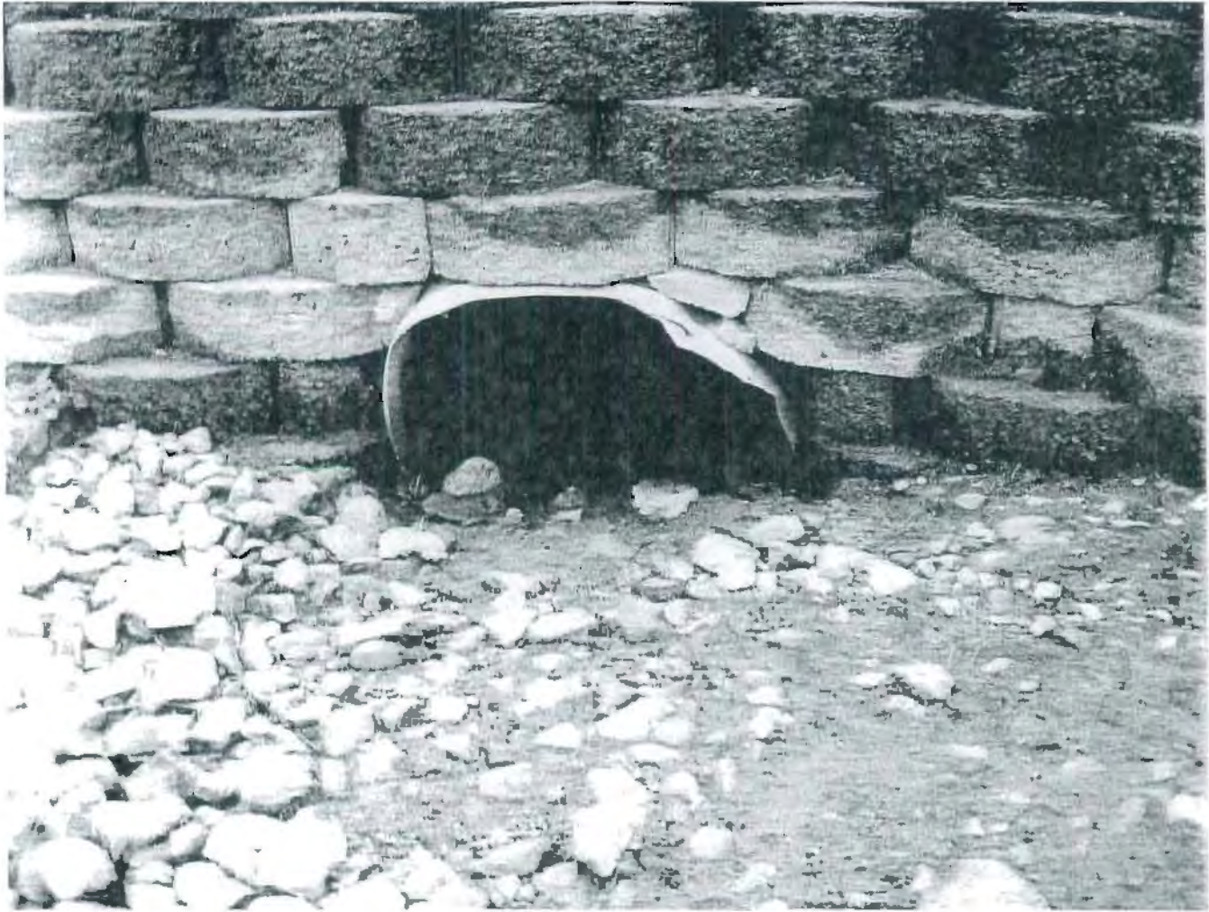
Photo 10 – Close up of culvert entrance
