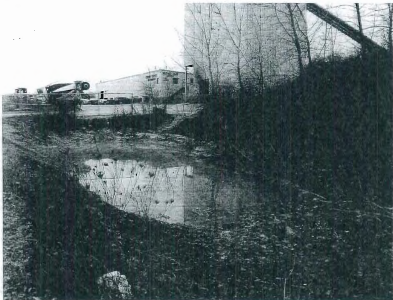
Photo 1 – Settling pond for concrete truck wash water adjacent to Spring Ridge Drive
