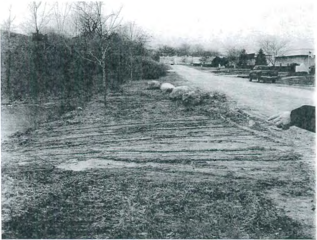
Photo 20 – indication that the basin may have been recently excavated to remove deposit build-up.
