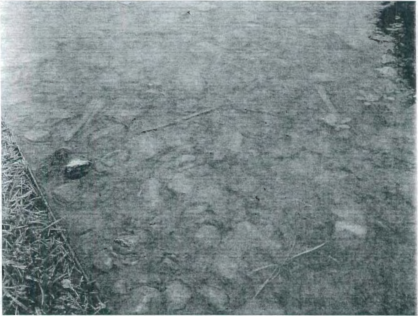
Photo 13 – Close up photo showing the deposits on the stones.
